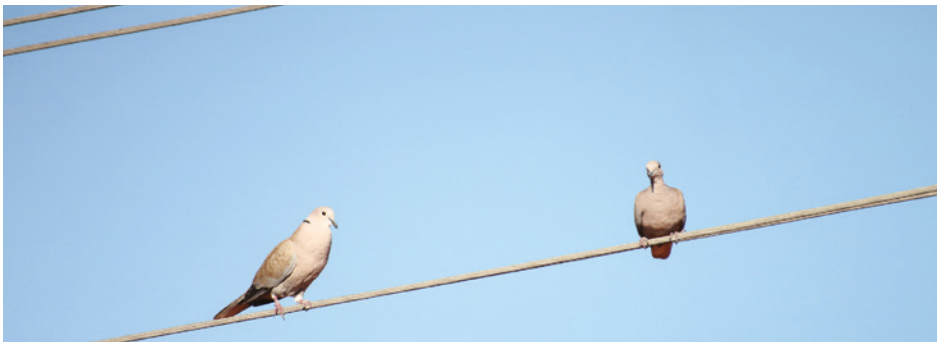
FIGURE 4.2.6 There is no potential difference between each bird’s feet.
